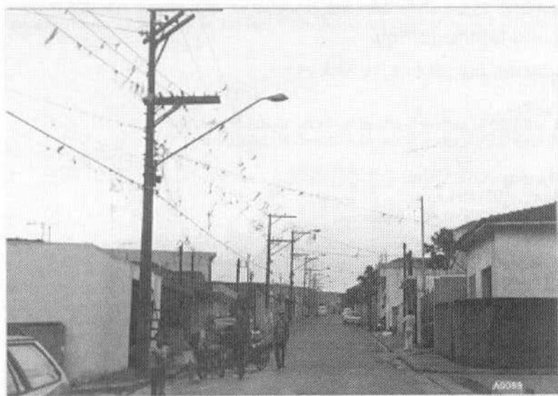
Fig. 2 Telephone wires and cables involved with kite strings.
